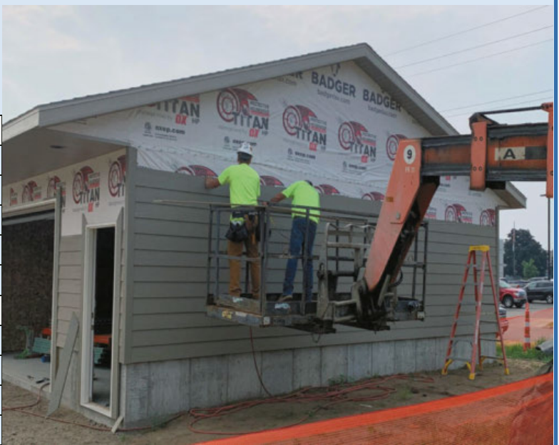
Pictured above & below: Fowler & Hammer carpenters work to side the shed addition.
