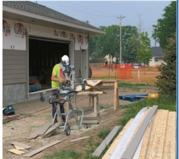
Pictured above & below: Fowler & Hammer carpenters work to side the shed addition.
