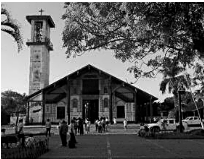
Cathedral of San Ignacio: Rebuilt in 2000 according to the original 1761 Jesuit church, conserving the 1967 intermediate cathedral bell tower which is presently being re-nodeled to harmonize with the rest of the Cathedral.
