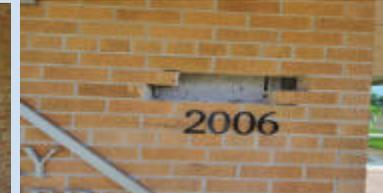
The most troublesome area has been the 2<sup>nd</sup> floor rectory walkout onto the roof (near the garage). The metal lintel has rusted – causing rust jacking, which puts stress on the grout, creates cracks, and allows water infiltration.
