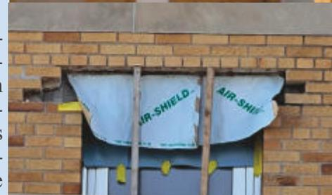
Replacing lintel and repairing damage of rust jacking
