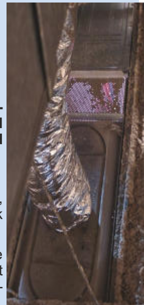
300 flex ducts in the attic are the source of fresh air circulation for church.
