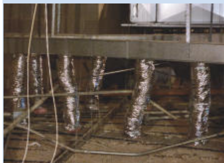
300 flex ducts in the attic are the source of fresh air circulation for church.
