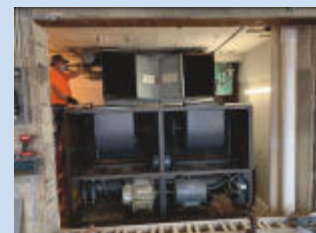
Dismantling the old air handling unit
